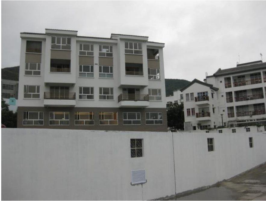
Part of the Shing Mun Springs complex
